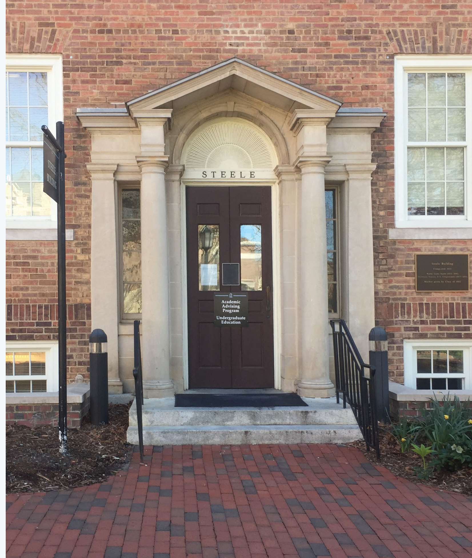
Steele Building, where the Carolina Women's Center was initially housed in the basement upon its establishment.
